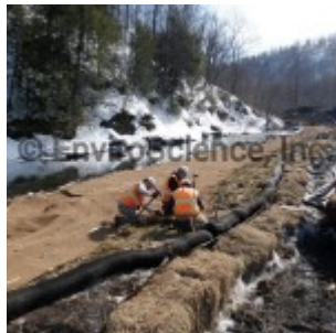
Soil stabilization and stormwater BMPs
