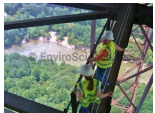
Preliminary Site Assessment
