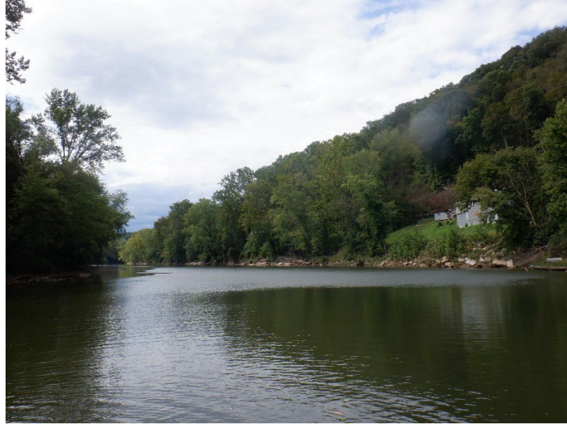
View of Elk River and failing streambank at the project location
