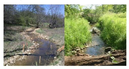
This design-build stream and wetland restoration enhanced 4.0 acres of wetland, created 2.53 acres of new wetland and raised stream bed elevations of two streams to reconnect 3,297 total feet of stream to its floodplain. This unnamed tributary in the headwaters of the Chagrin River watershed had been channelized in the past to drain adjacent agriculture properties, and had become entrenched.
